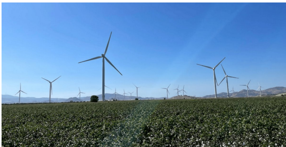
FIGURE 8: Field view of the proposed WPP project location in Bergama
