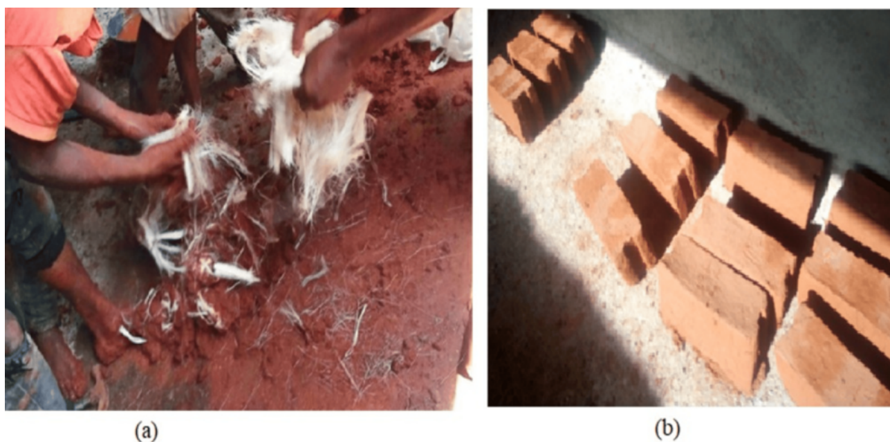
FIGURE 6: Fiber mixing (a), molding and curing (b) of adobe blocks
